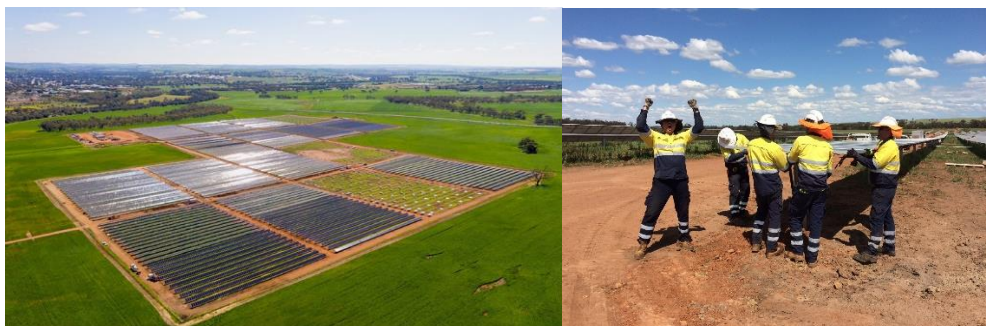
Northam Solar Farm in September 2018 (left) and construction team finishing the last panel (right)
