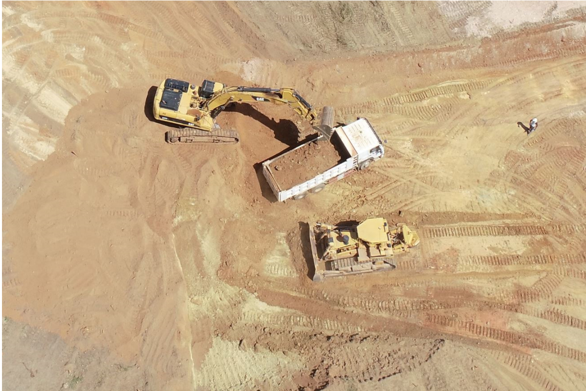
Photo 2: Box cut establishment
