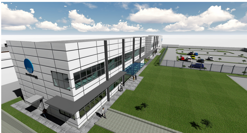
Figure 3 – Administration and Process Building
