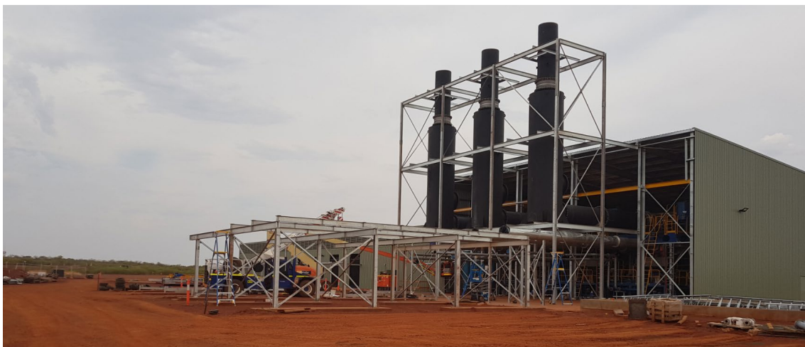
Dead Bullock Soak Power Station exhaust system under construction at Newmont Mining Corporation's Tanami Operation.
