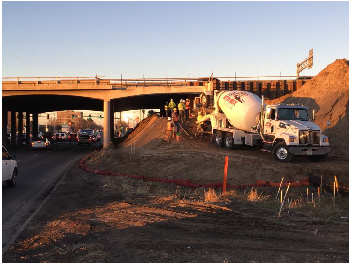
Figure 2. EdenCrete® shotcrete mix being supplied to the Project
