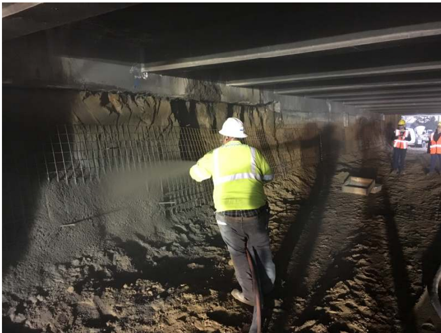
Figure 1. EdenCrete® shotcrete concrete mix being applied
