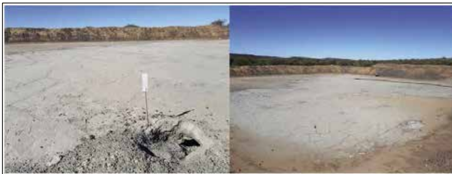
Figure 4-16: Reid's Ridge tailings dam with Auger holes, Warriedar project
