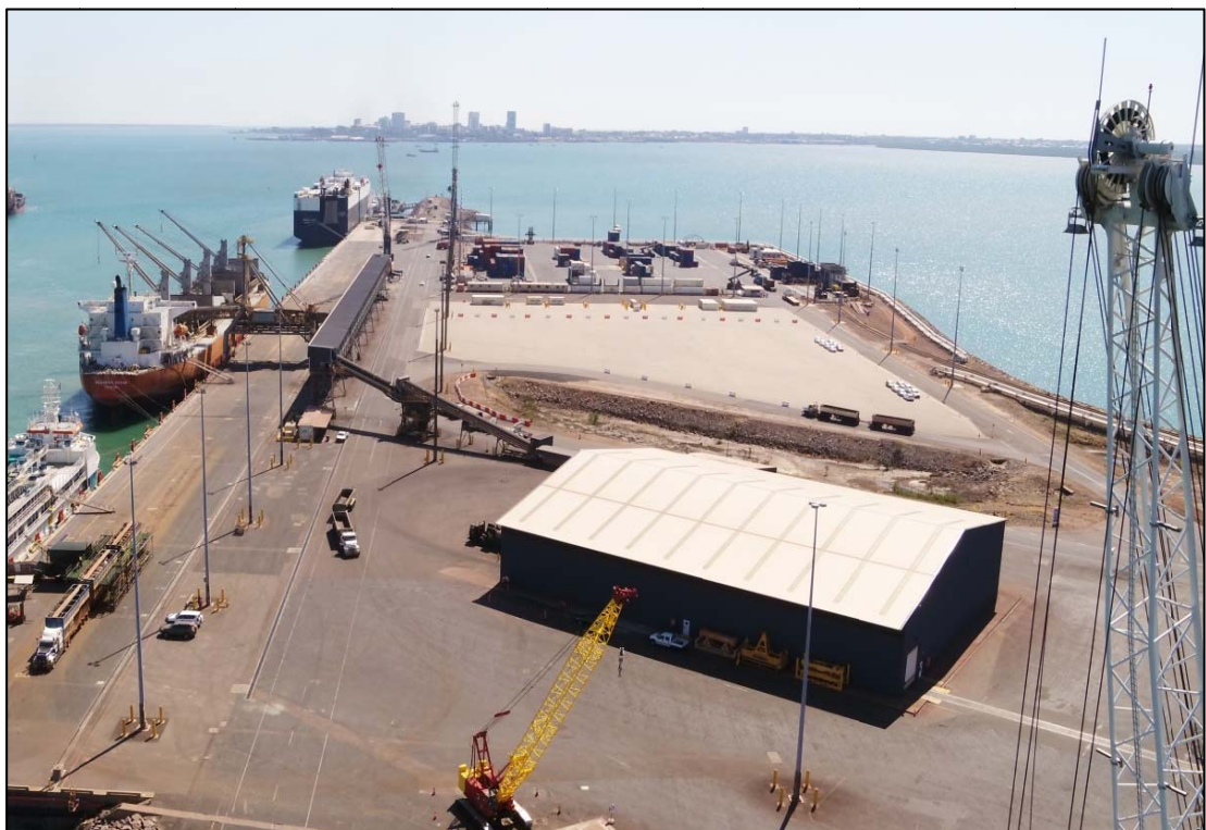
Figure 2 Darwin Port loading facilities (travelling gantry and autoloader)
