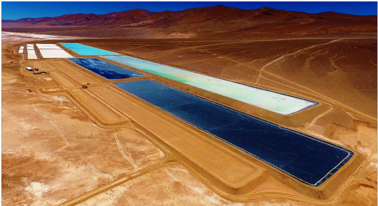
Figure 1. Rincon Lithium Project – Additional Stage Evaporation Ponds Constructed
