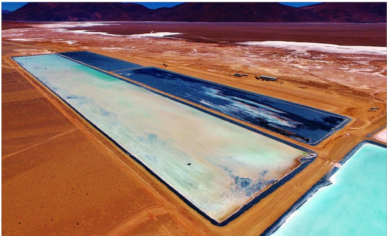
Figure 2. Rincon Lithium Project – Additional Stage Evaporation Ponds Constructed
