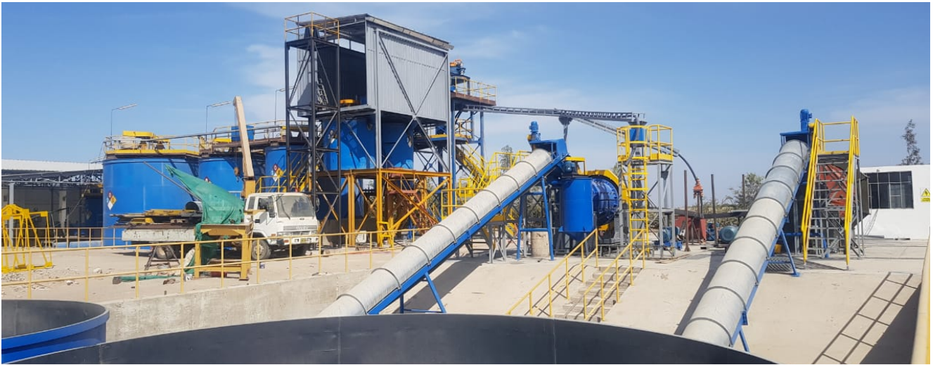
Figure 2 | View of Vista Gold Plant grinding circuit (right) and CIP processing (left) from fine ore feed bins in the foreground
