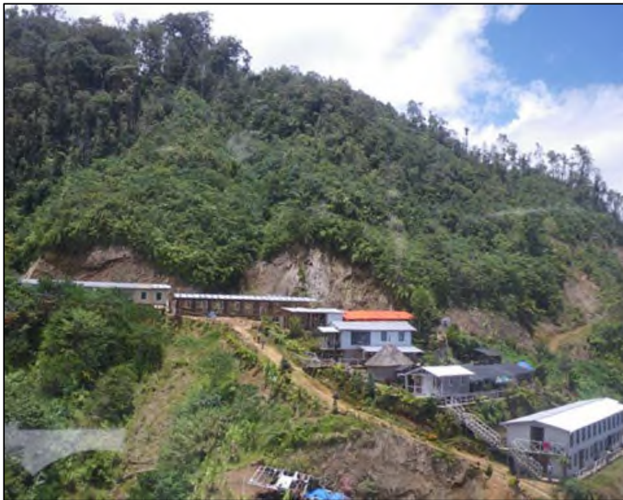
Crater Mountain Site Office and Accommodation, Sept 2016
