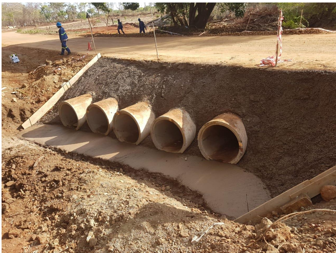
Figure 4: Access Road Culvert Construction
