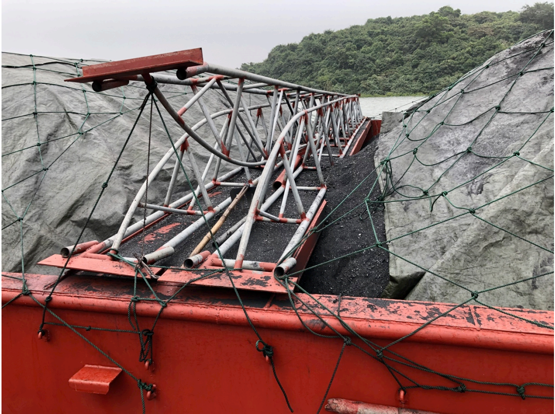
Relocatable Access across Barges
