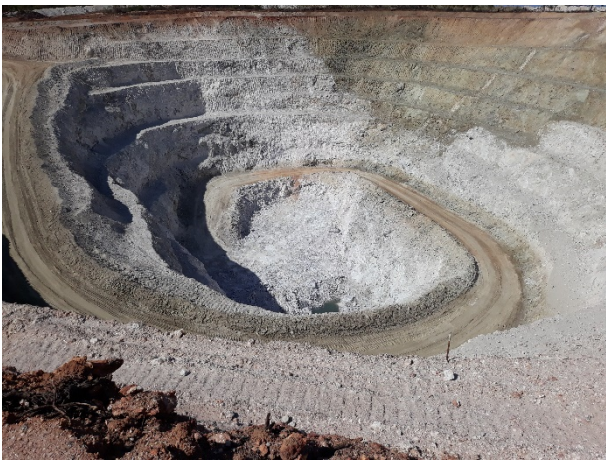
The completed Sinclair Stage 1 Pit
