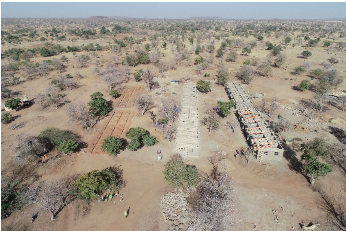
Photo 3: Stage 1 Camp Area
