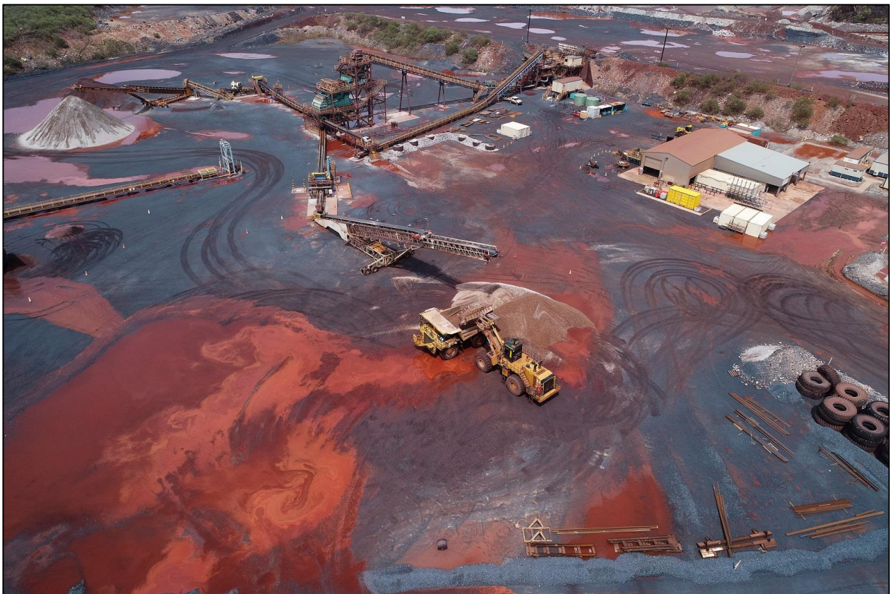
Figure 4: Crusher recommissioning, January 2019.
