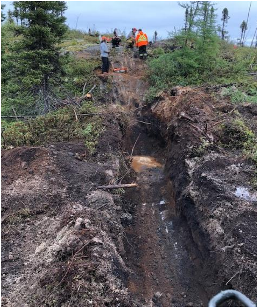
Figure 3: Trenching and sampling being undertaken at the Lac Rainy Graphite Project, Quebec
