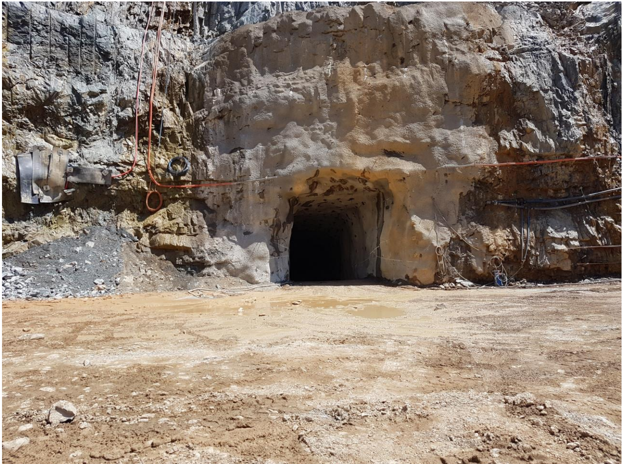
Main decline portal in Wyoming One pit
