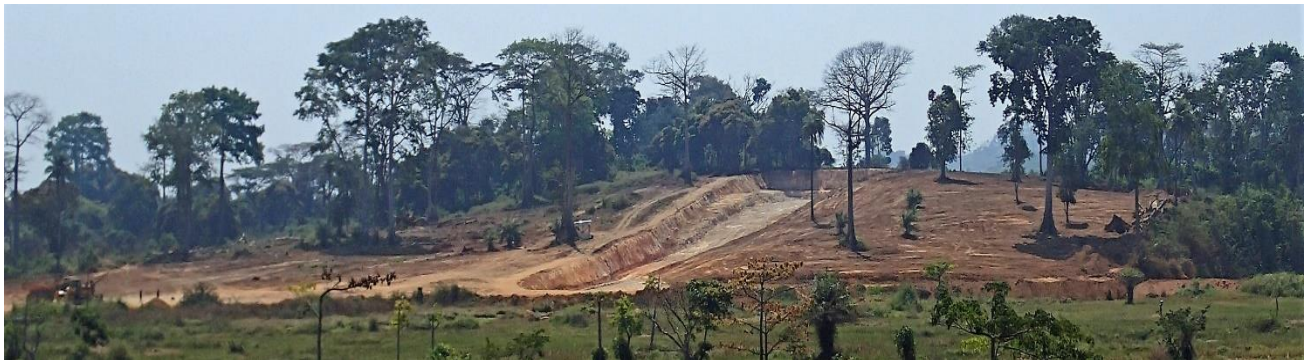
Figure 1: Partially excavated Boxcut at the Tongo mine
