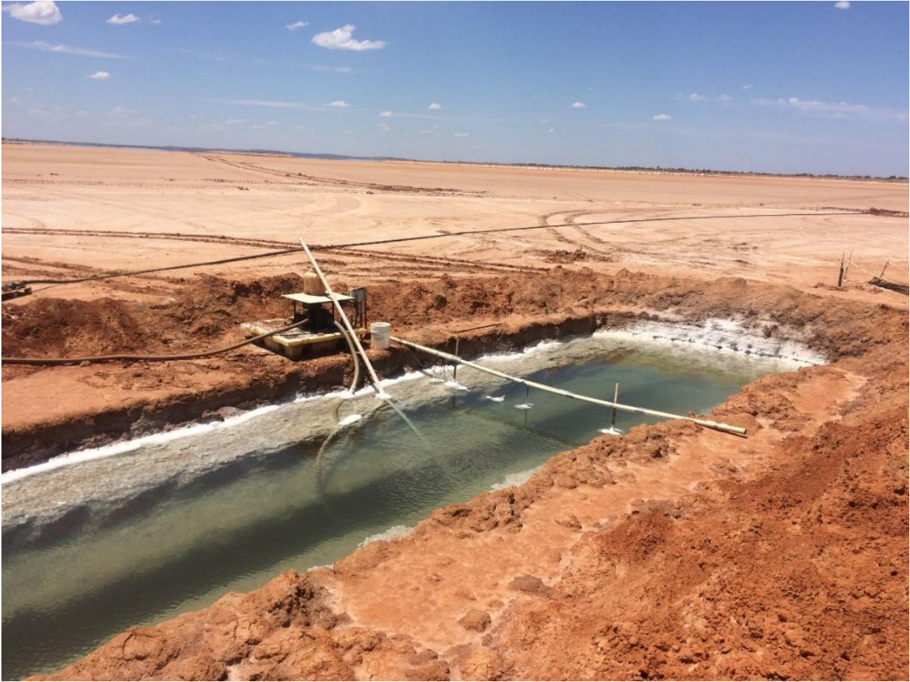
Figure 11: Lake Ballard trench and pump setup
