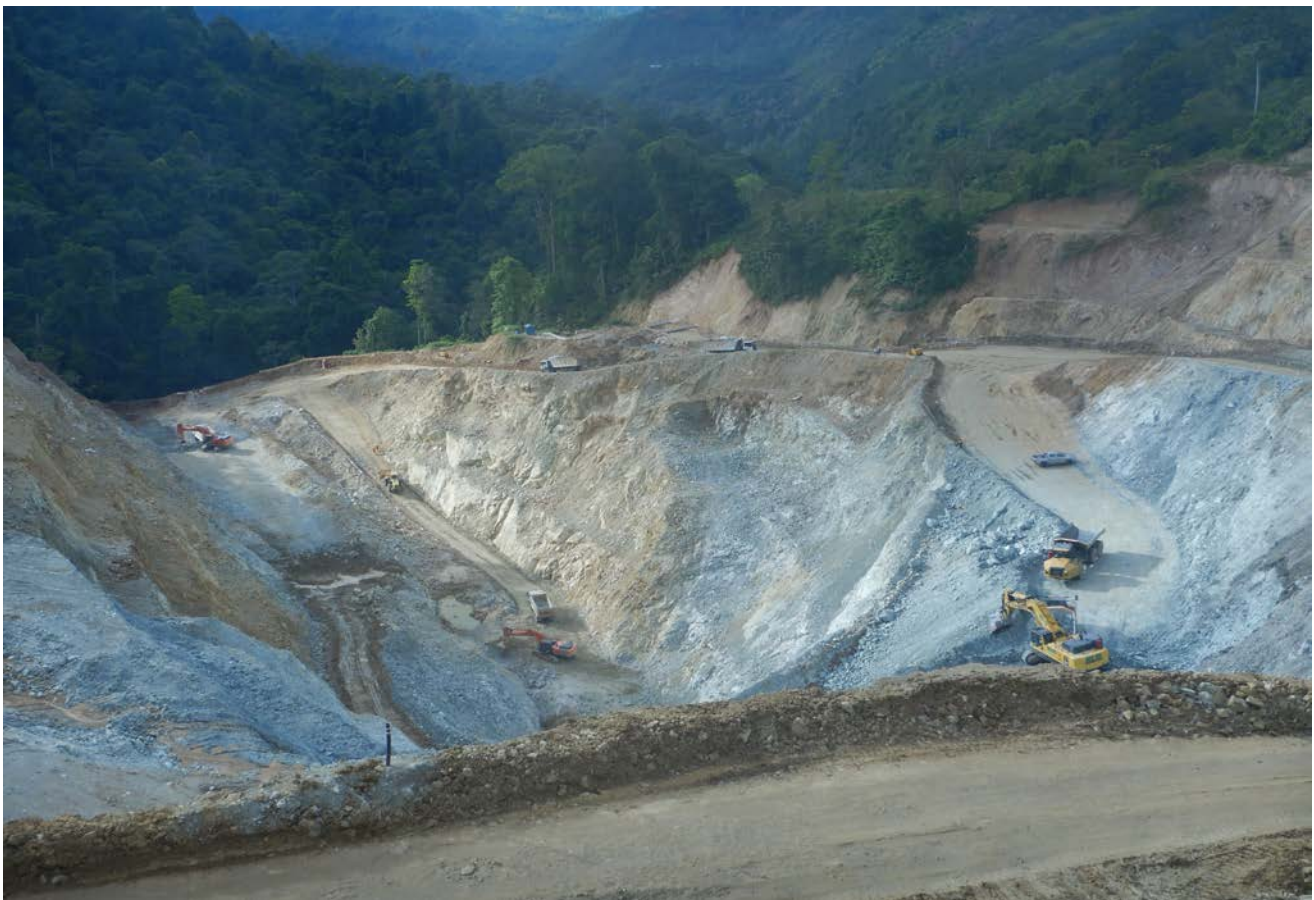
Figure 1: Way Linggo Open Pit at 31 December 2018, looking south
