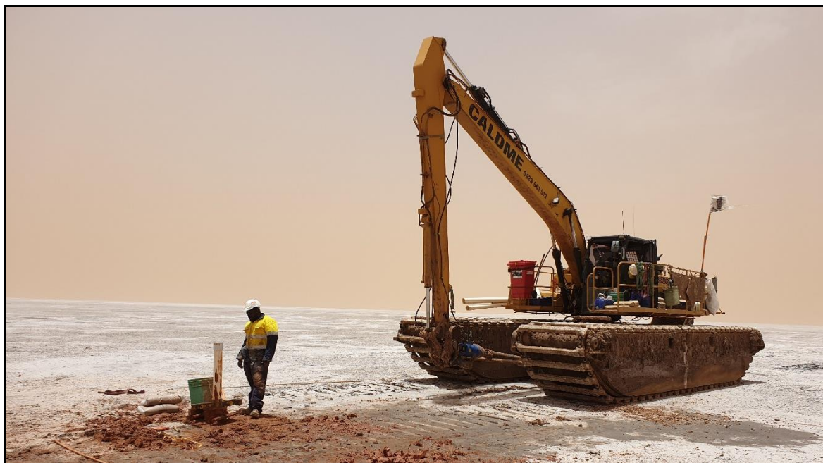
Figure 4. A completed bore
