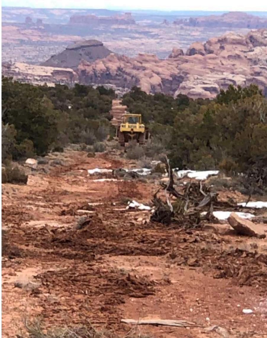
Photo 2: Roadworks in progress to upgrade access to the Skyline Unit 1 well.
