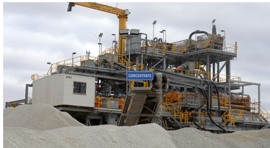
Bald Hill DMS Plant
