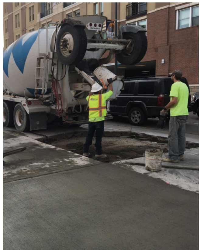
Figure 2. EdenCrete® Trial Slabs in first trials.
