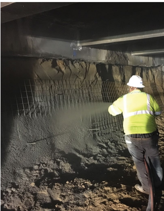
Figure 1. EdenCrete® shotcrete concrete mix being applied
