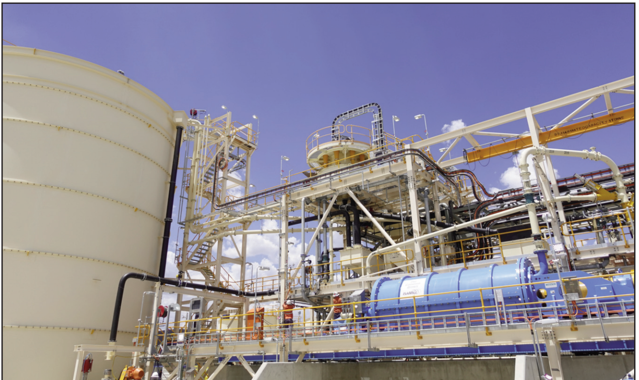
Figure 5: IsaMill™ installation - finalising piping and electrics
