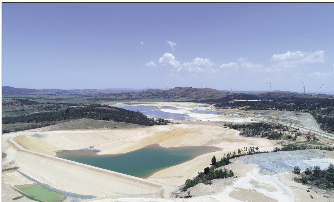
Figure 7: Tailings Storage Facility 4 - stored water for the commencement of wet commissioning. View to south – area of tailings mining in the background.
