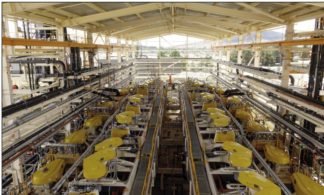
Figure 6: Flotation building - finalising piping and electrics
