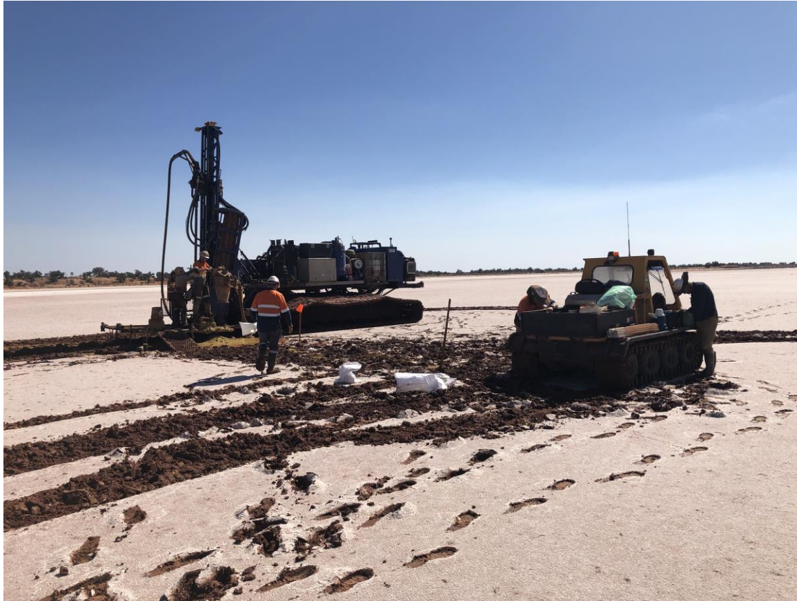
Lake drilling – Jan/Feb 2019
