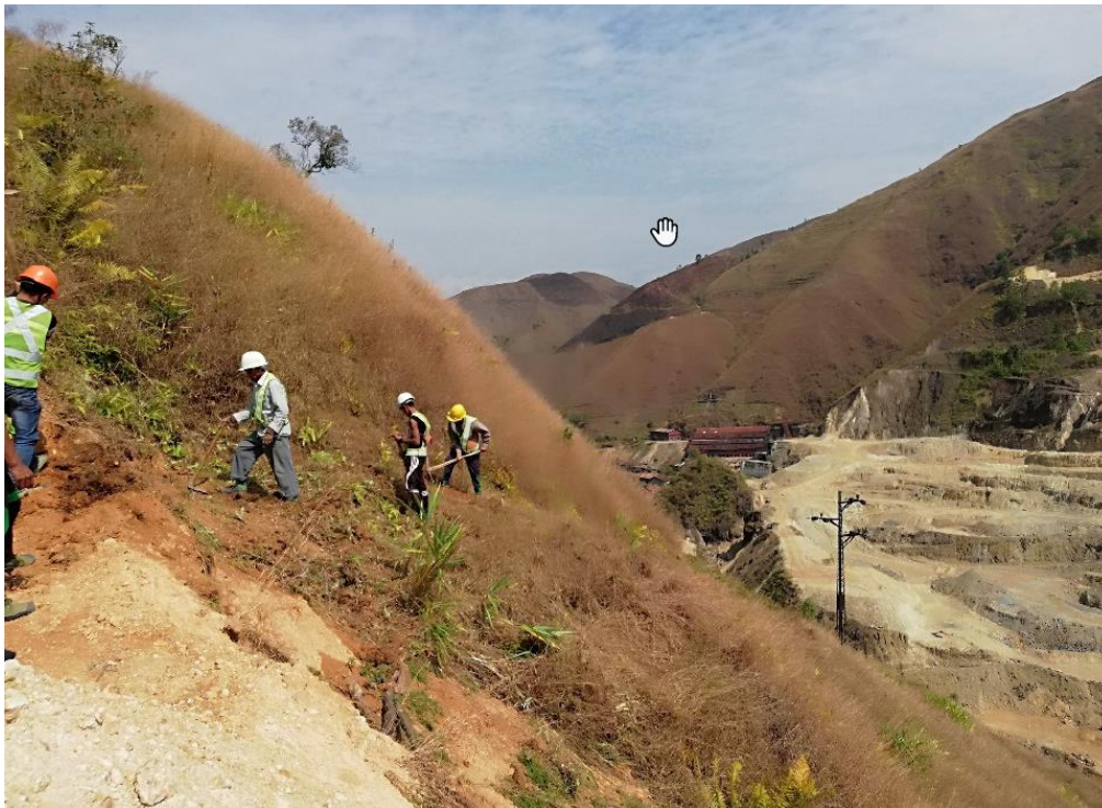
Figure 8. Photo, looking northwest showing commencement of Yegon Ridge access for man-portable drilling rig.
