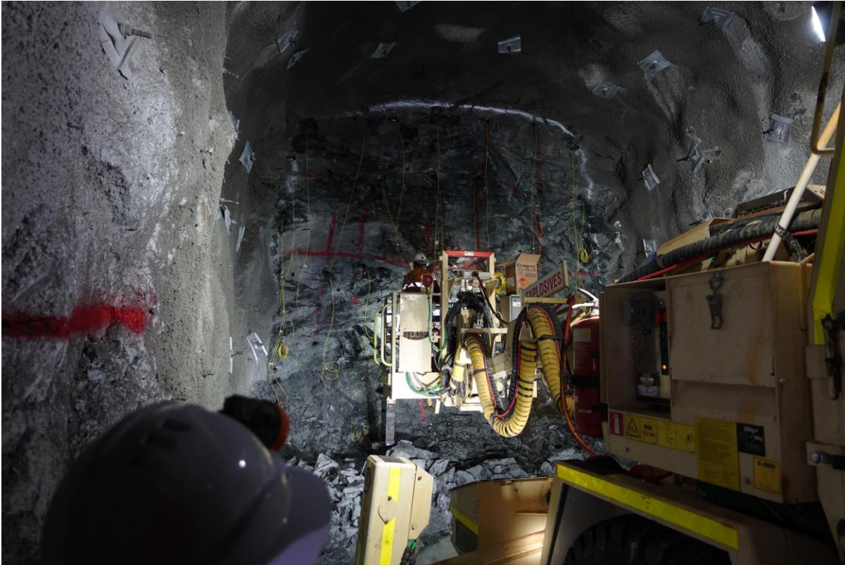
Figure 1 Underground Mining Operations
