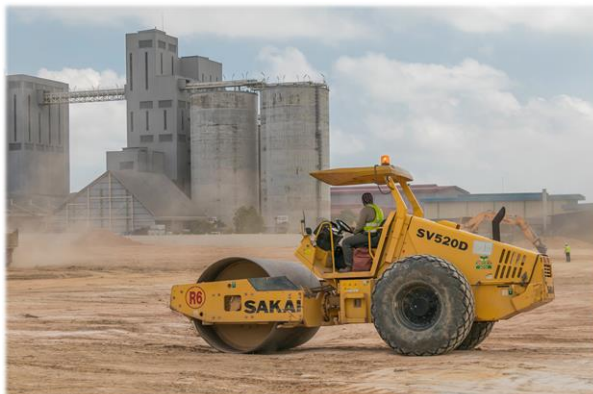
Compaction of site to specification
