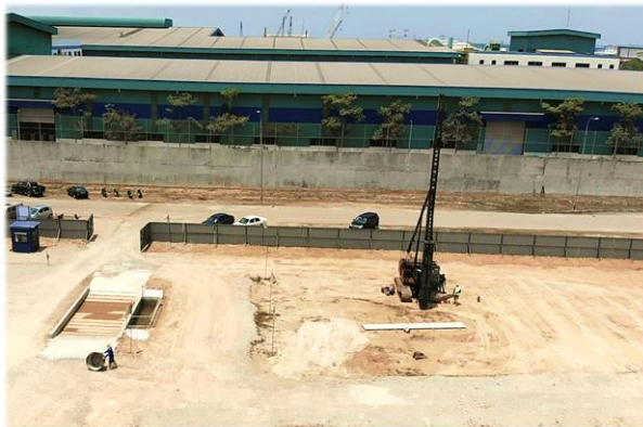
Foundation piling rig on site for tests
