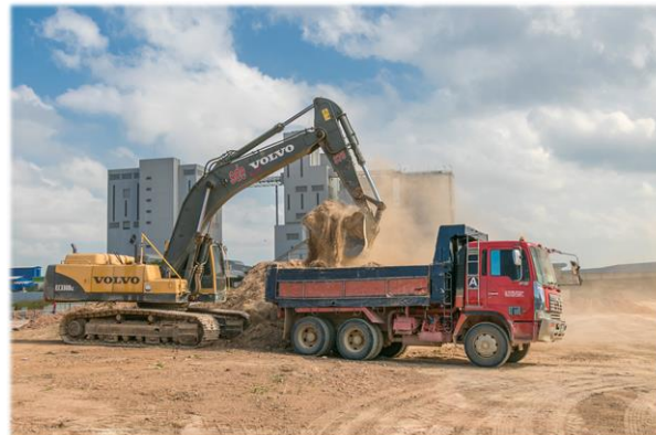
Top soil removal completed
