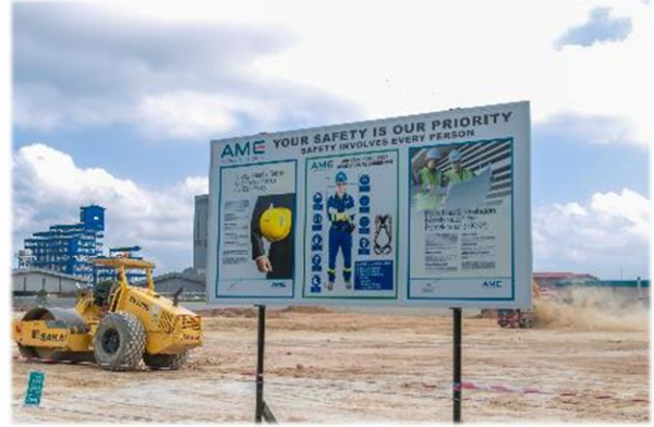
Site safety procedures established
