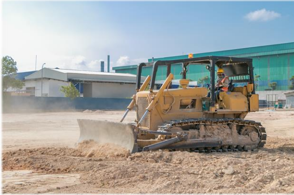
Bulk earth works and leveling
