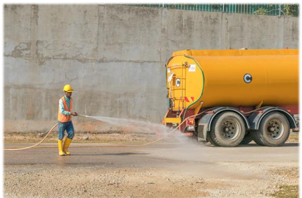
Watering and compaction of site
