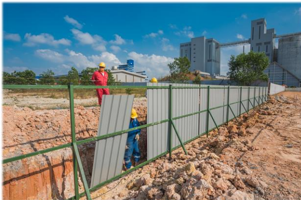
Completion of site perimeter fence
