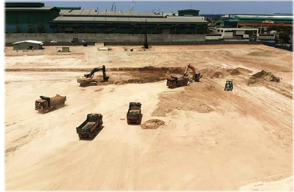
Bulk earthworks and soil removal
