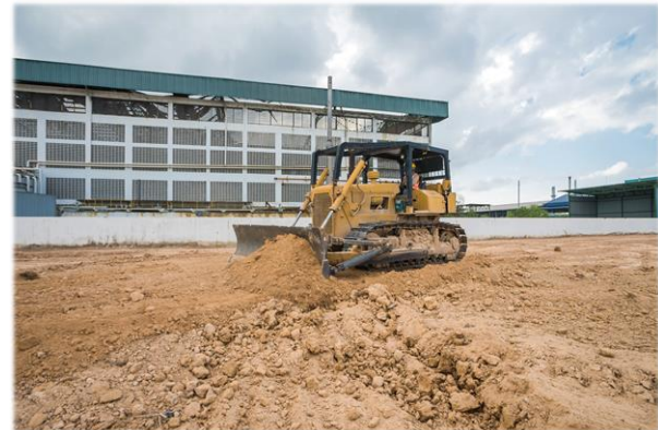
Site leveling to specification
