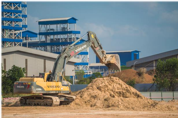
Top soil removal completed
