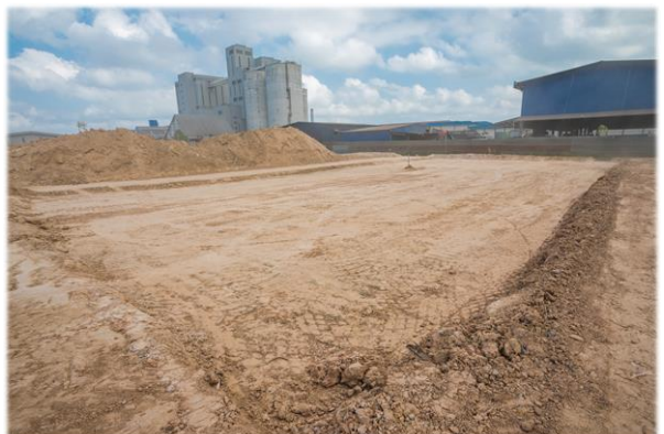
Compacted workshop pad
