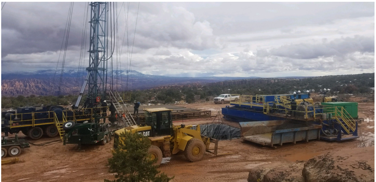
Figure 1: Long Canyon No. 2 well pad with work over rig in operation
