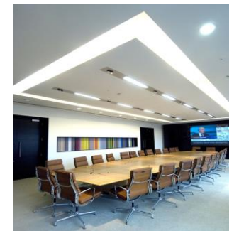
Office LED Lighting
