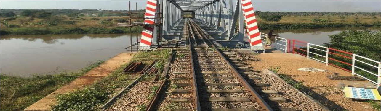
Figure 3: Typical steel bridge on the Camrail line.
