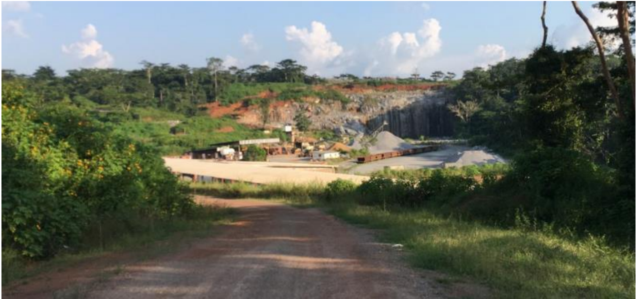
Figure 4: Camrail quarry supplying track ballast & concrete aggregate for manufacturing track sleepers.
