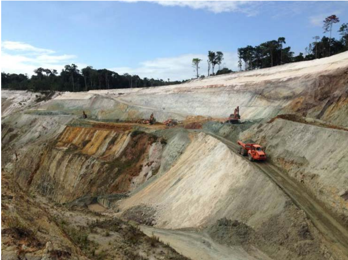
Figure 1: Progress on Smarts 3 pit Cutback.
