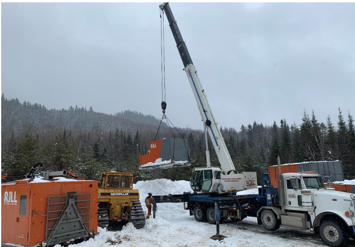
Figure 1: Diamond drill rig being set up at the first drill site at the Lac Rainy Graphite Project
