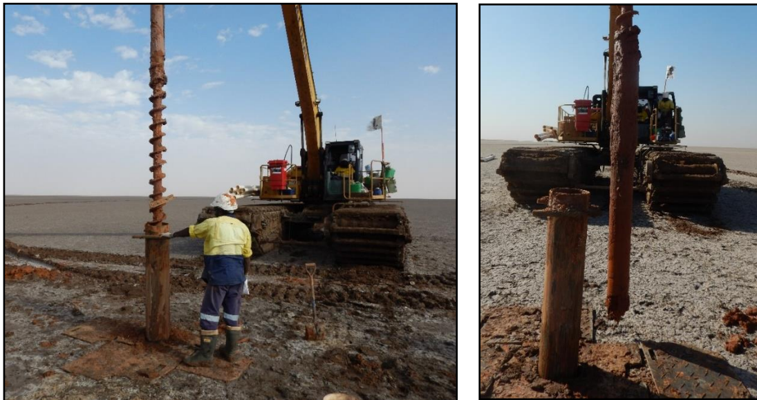
Figure 7. Auger Drilling with Surface Casing
