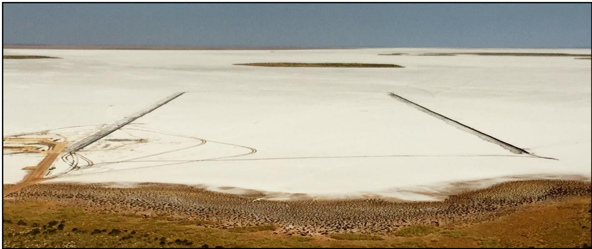
Figure 4. The 1 kilometre brine extraction trenches, September 2017
