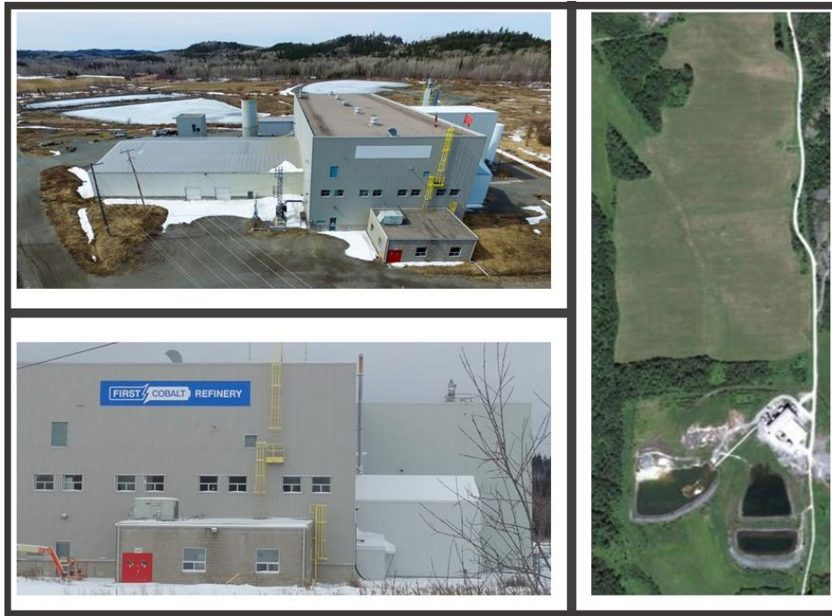
Image 3. Exterior and property footprint of the First Cobalt Refinery
