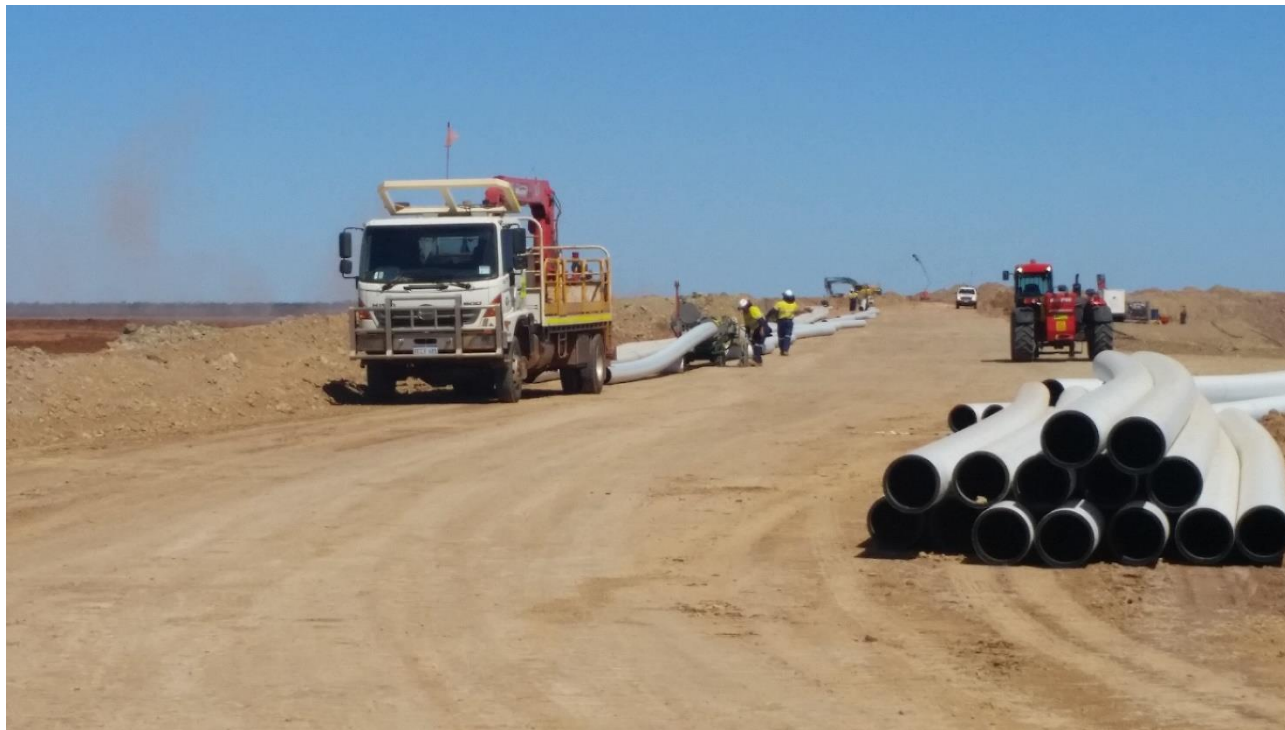
Figure 3: Preparation of pipeline for dewatering of the Williamson Pit brine
