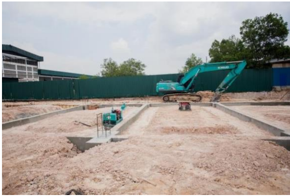
Building concrete footings
