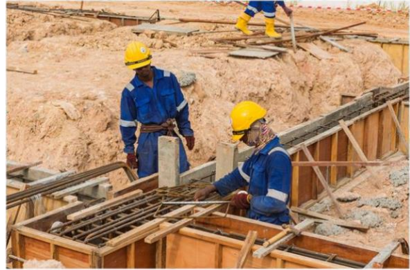
Building civil footings
