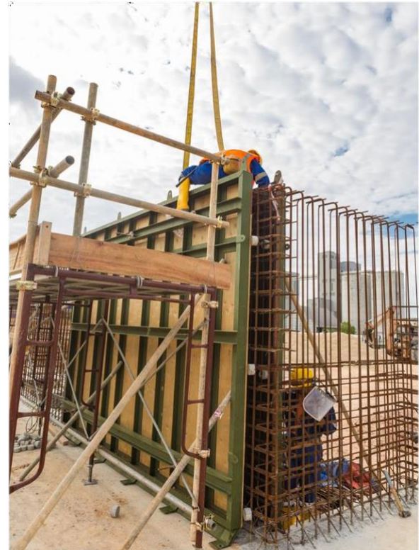
Steel work for concrete retaining wall
