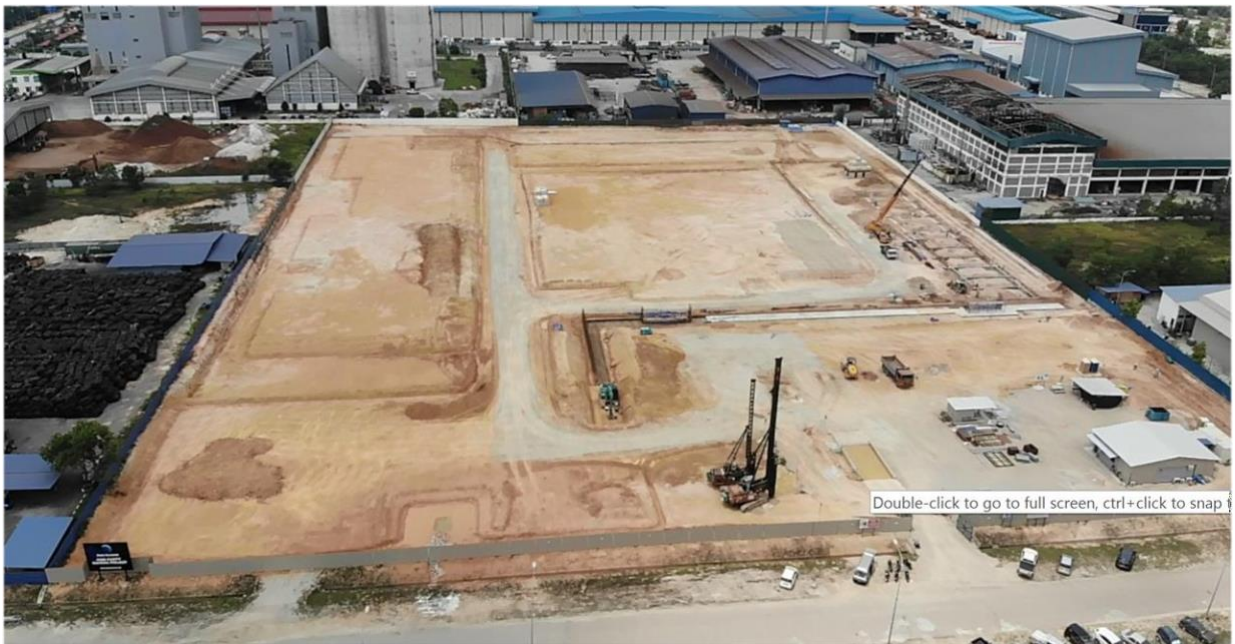
Aerial view showing progress of Stage 1 construction
