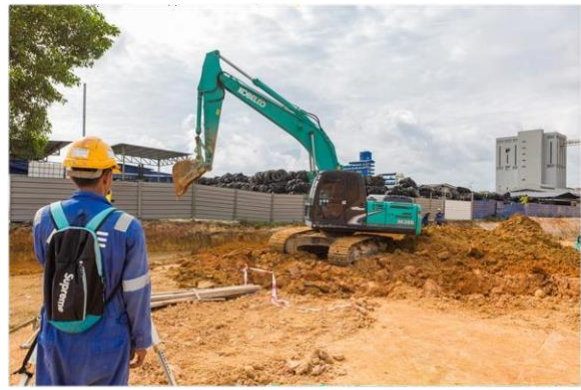
Workshop building ground works
