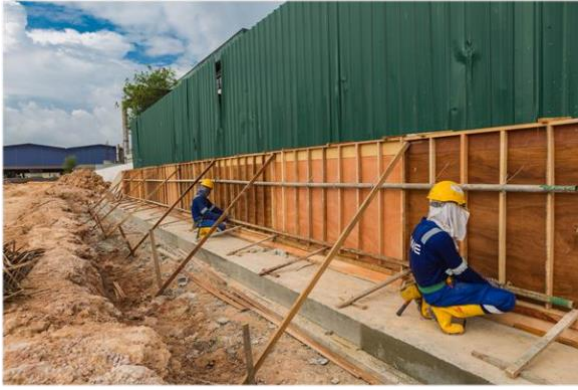
Boundary retaining wall
