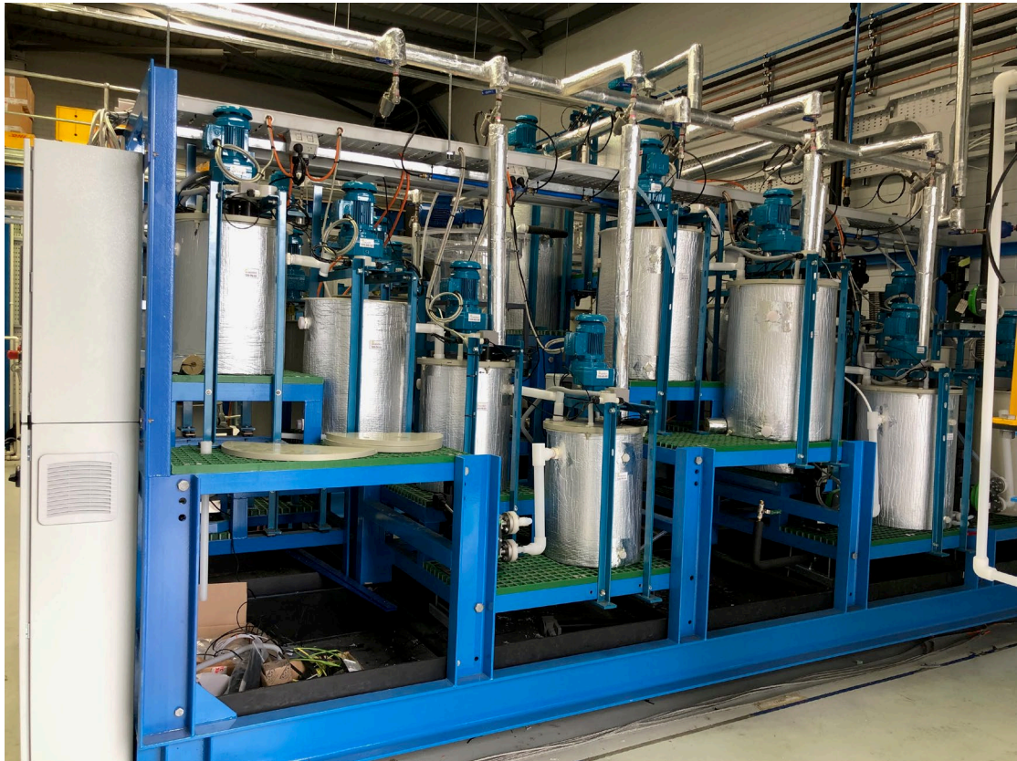
Figure 3. Leach skid: electrical installation complete and wet commissioning in progress 15 April 2019.
