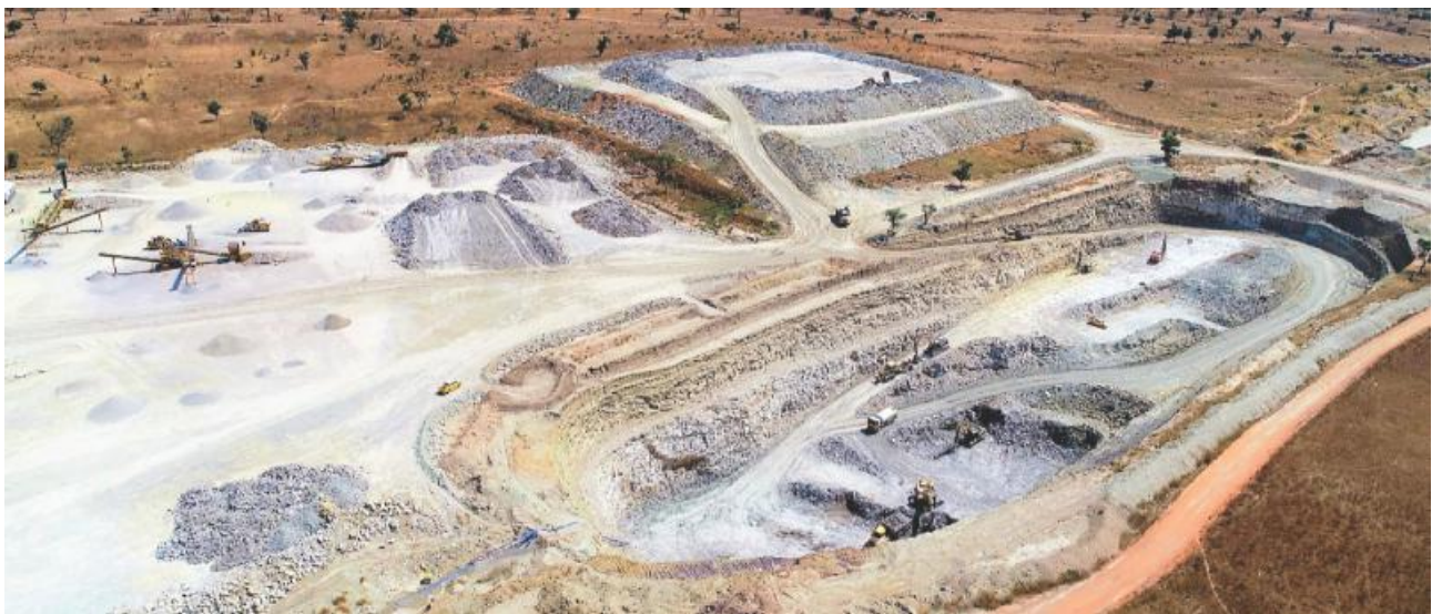
Figure 10. Macy Mine Pit and ROM Pad
