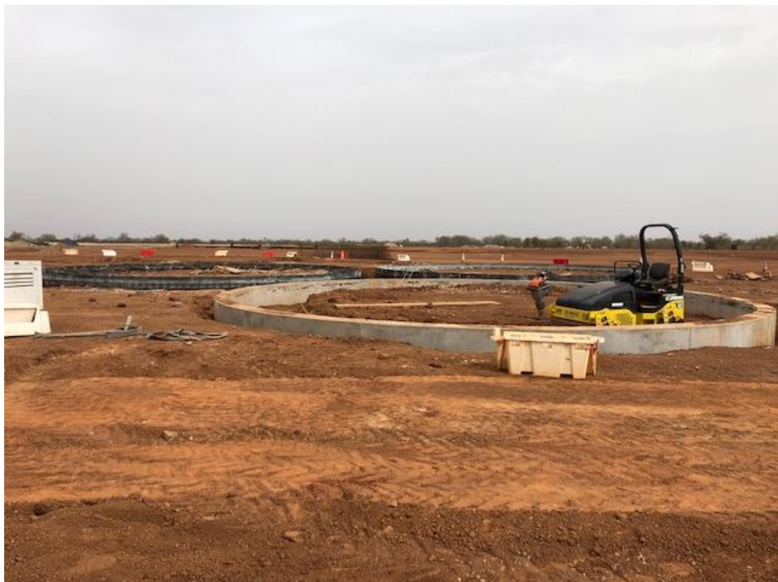
CIL Tank Ring Beams Following Concrete Pour
