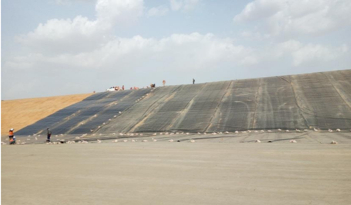
WSF HDPE Liner Installation
