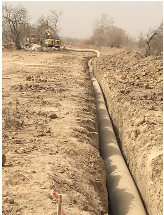
Water Pipeline Trenching and Placement
