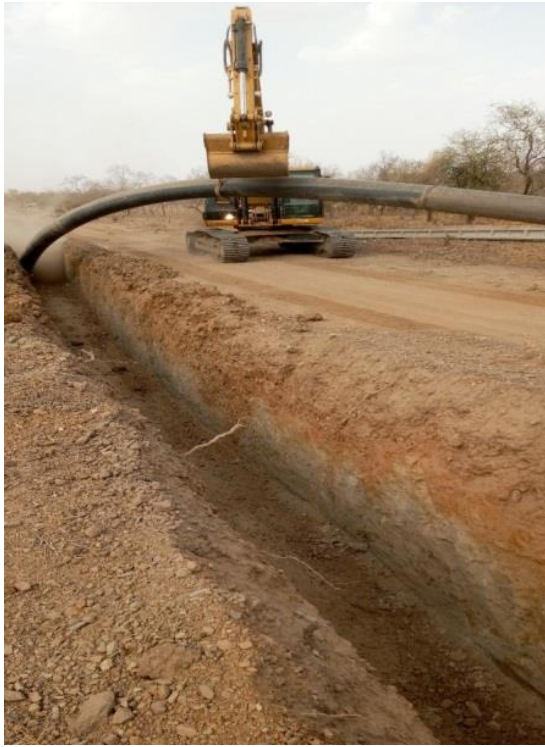
Water Pipeline Trenching and Placement
