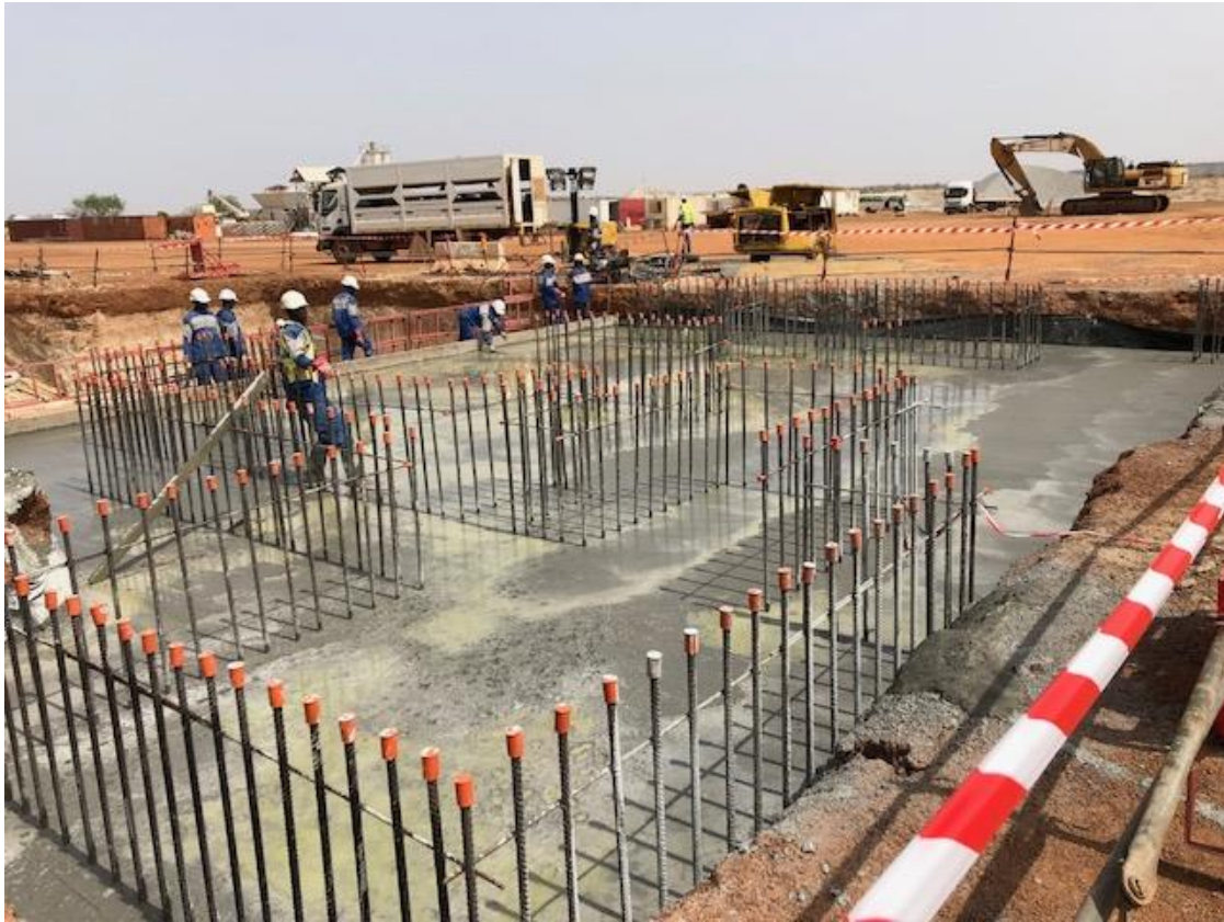
SAG Mill Foundation following First Concrete Pour
