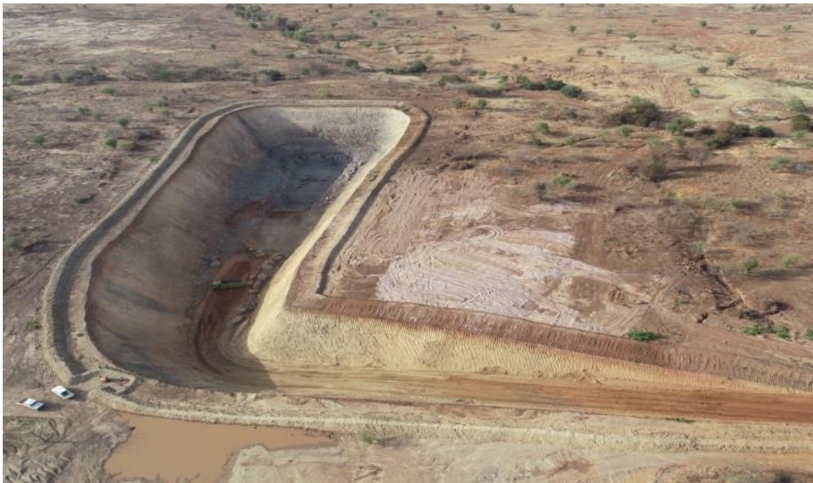
Underground Access – Boxcut Nearing Completion
