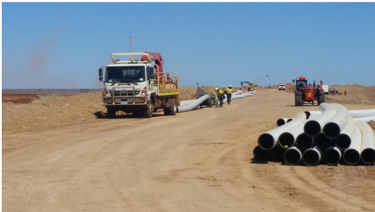
Figure 8: Preparation of pipeline for dewatering of the Williamson Pit brine
