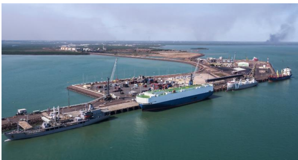
Figure 3: Darwin Port, East Arm Wharf.
