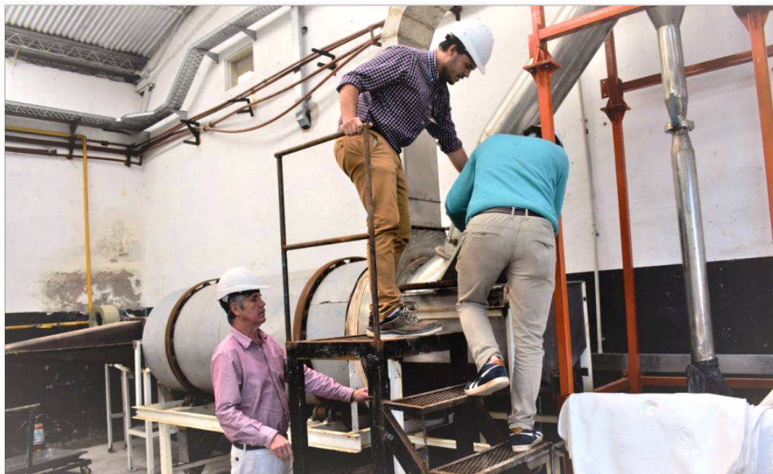
Figure 1. Rincon Lithium Project – Preparation for Continuous Pilot Plant Processing Works
