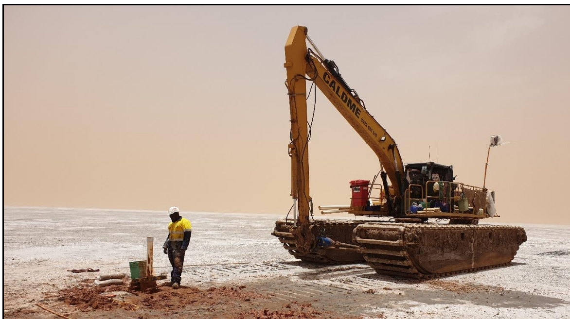
Figure 3. A completed bore
