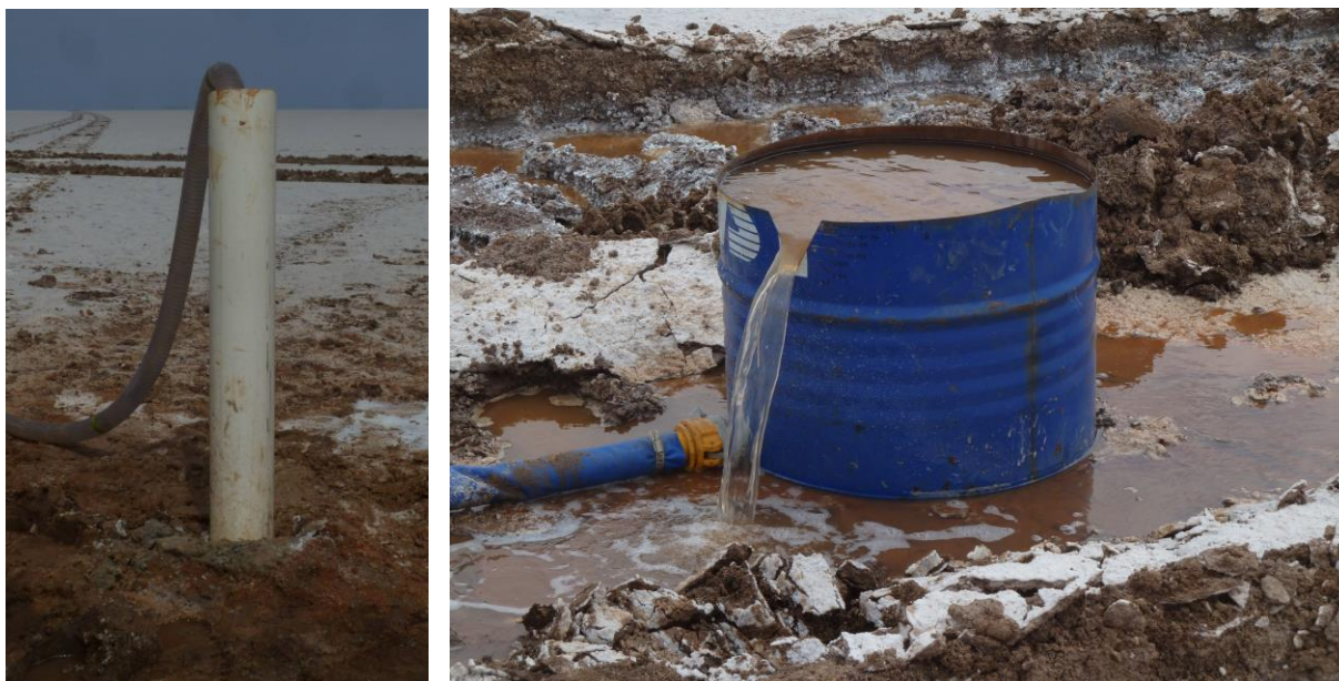
Figure 4. Bore development with pump flow rates recorded by a V-notch weir
