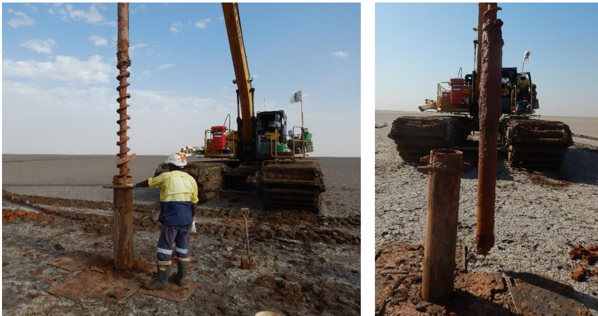
Figure 2. Auger Drilling with Surface Casing
