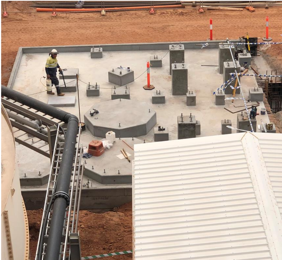
Figure 7. Concrete pad area and plinths nearing completion in preparation for mill installation
