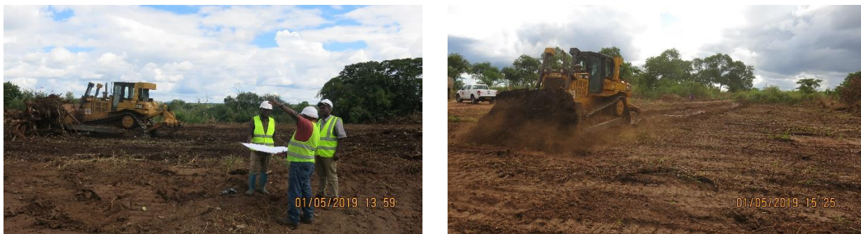
Figure 4. Photos of current activity on site at Lindi Jumbo Graphite Project.
