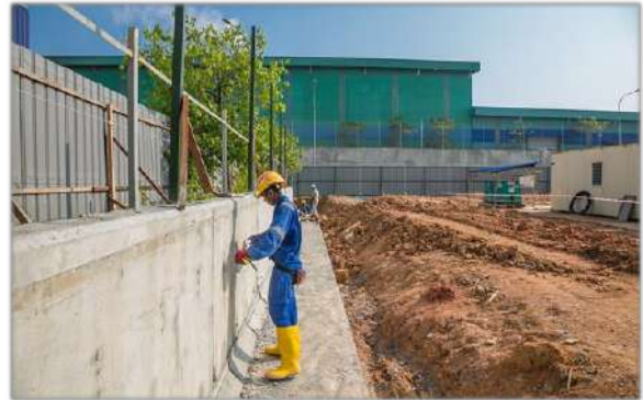
Boundary retaining wall
