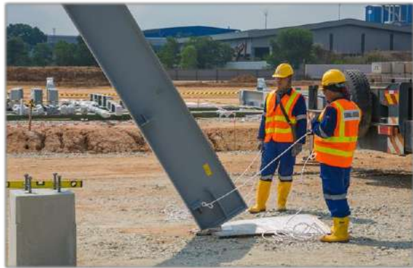
Local rigging contractors
