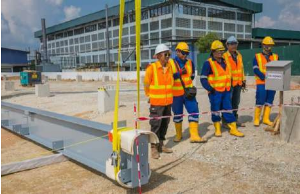
First steel column ready for lift
