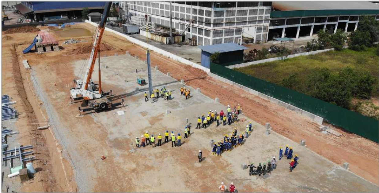
Erection of the first maintenance workshop column
