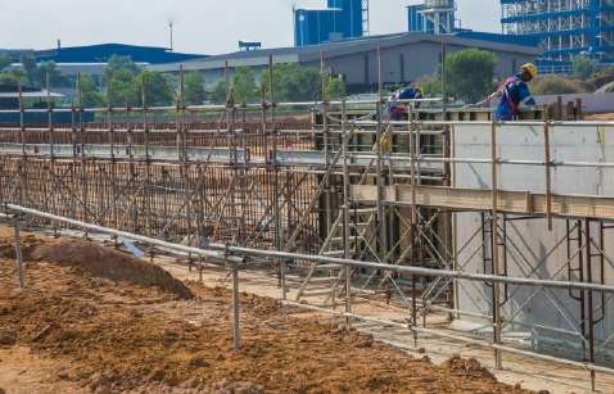
Administration building retaining wall
