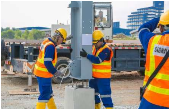
Securing the first steel column
