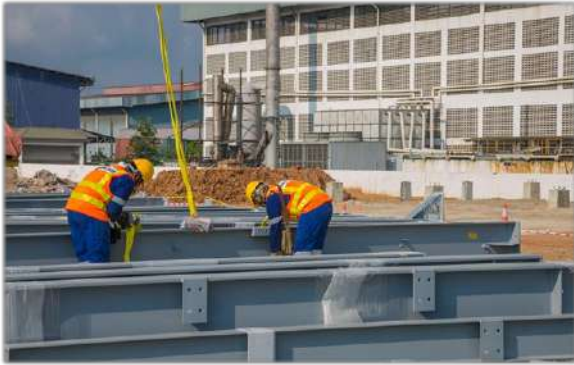
Delivered steel with quality control
