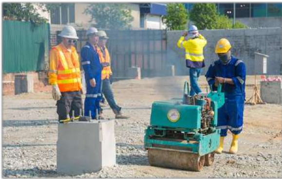
Concrete footings of workshop building
