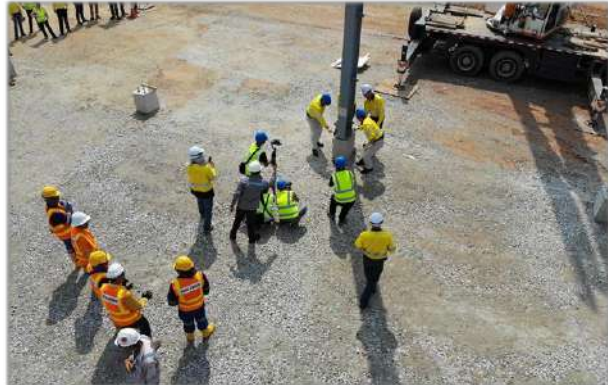
Securing the bolts
