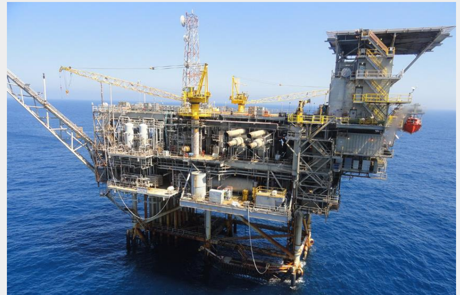
Green Canyon 18A Production Facility
