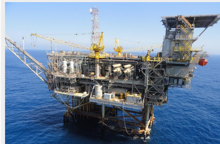
Green Canyon 18A Production Facility
