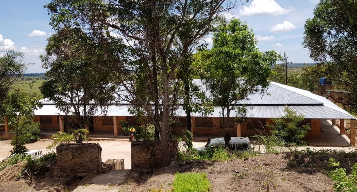
Image of the Refurbished Office Complex at Site
