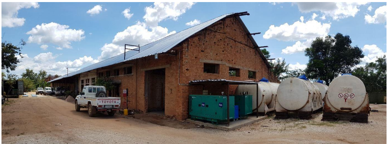
Refurbished Core yard and logging facilities including diesel storage tanks (100,000lts capacity)
