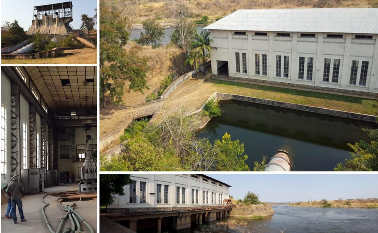
Images of the Piana Mwanga 32Mw Hydro Facility
